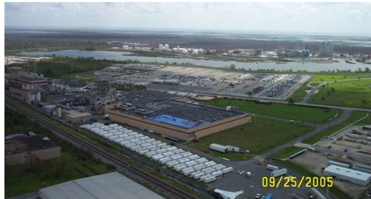
Trailer village for employees at the Gentilly plant
