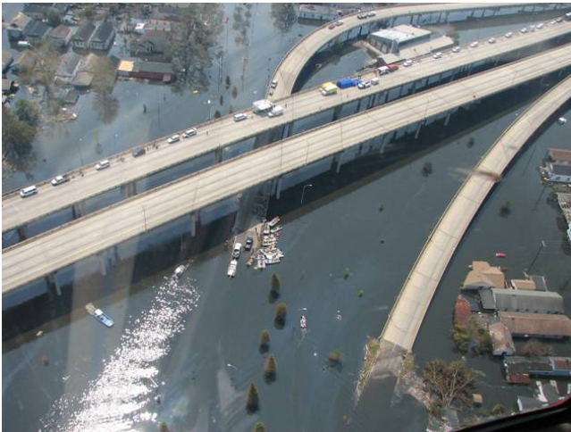
Access roads destroyed
